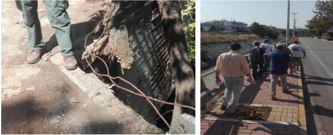
Figure 10 Identified spot hazard (unprotected edge), near Varymbombi at northern Attica (left); Small pedestrian adjacent to the river bank (elevated) and road, near Filadelfeia at southern Attica (right).
