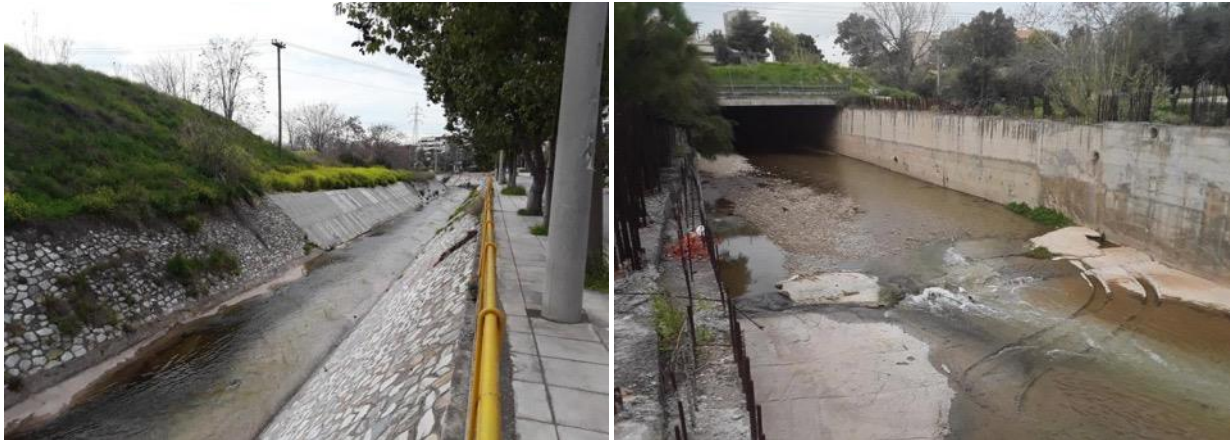
Figure 2 Change from stone built to concrete river bank coating (left), and transition from natural to engineered channel bottom (right).
